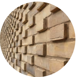
Type 8: Projecting Feature Brickwork
