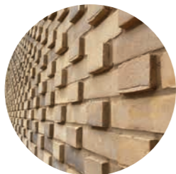
Type 8: Projecting Feature Brickwork
