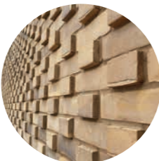
Type 8: Projecting Feature Brickwork
